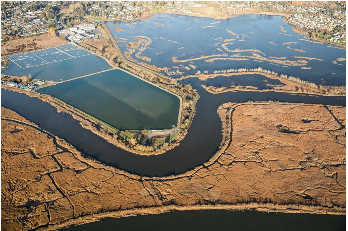
Aerial view of Puget Sound. © UW Climate Impacts Group, with aerial support provided by LightHawk.
