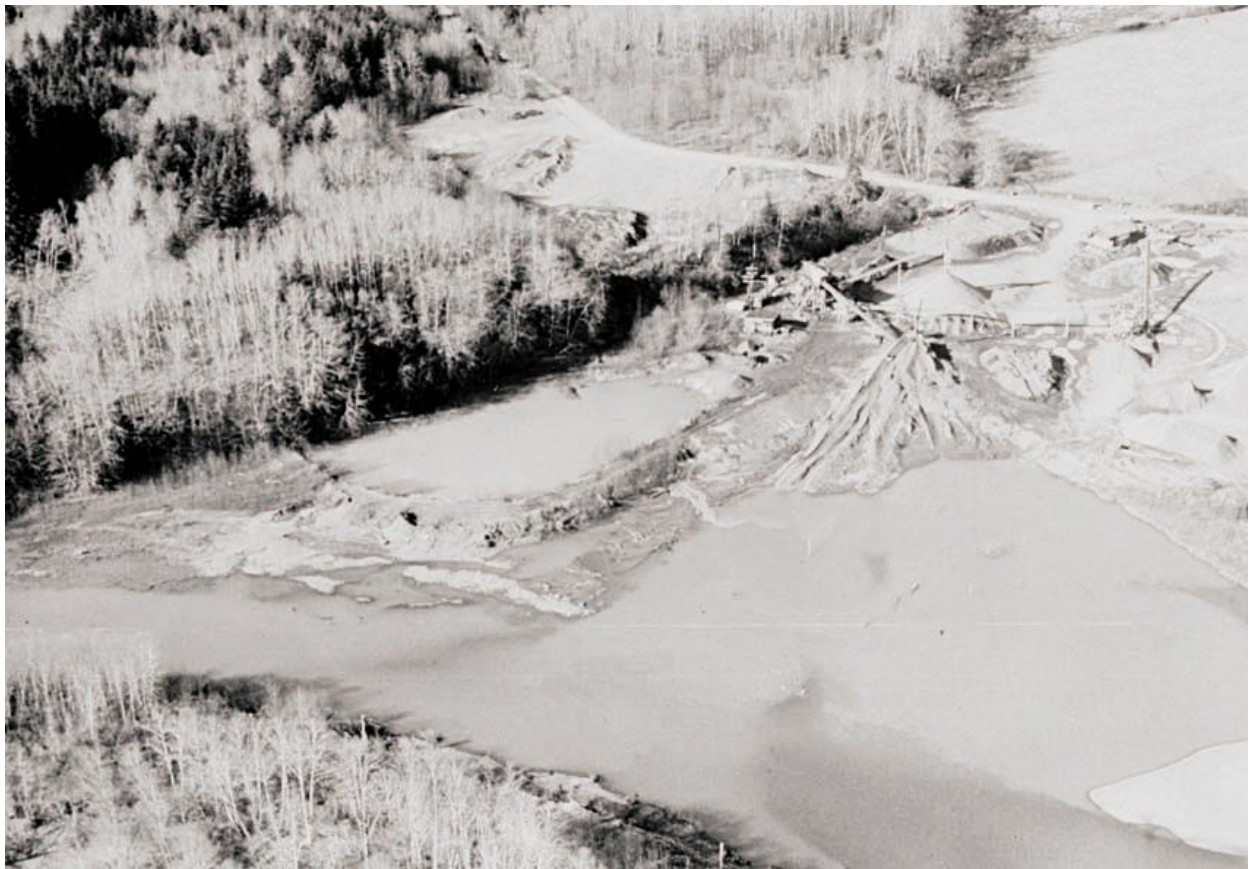
A gravel mine on the Wynoochee River, Wash. in 1965 that was created by gravel bar removal and shoreline mining. These types of mining techniques are no longer practiced in Washington. Evidence of turbid water discharge from the sediment pond to the river can be seen at the center of the photo. Photo: Lloyd Phinny, Washington Department of Fisheries.
